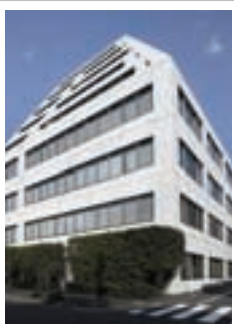
A-32 KDX芝大門ビル KDX Shiba-Daimon Building
