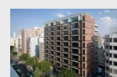
KDX Nagoya Sakae Building
