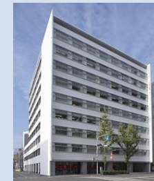
KDX Hakata-Minami Building
