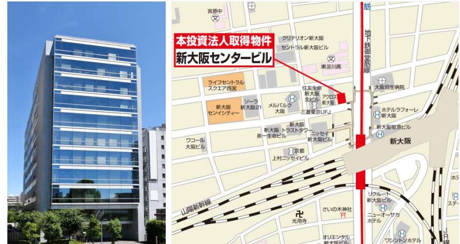
Shin Osaka Center Building
