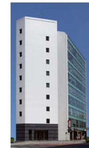
A92 Akihabara SF Building
