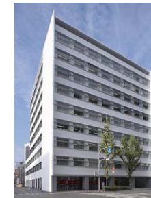
A53 KDX Hakata-Minami Building
