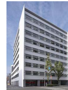
A53 KDX Hakata-Minami Building
