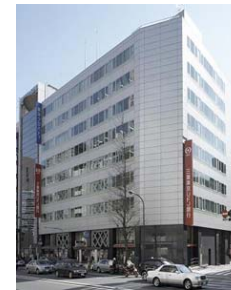
A40 Toranomom Toyo Building
