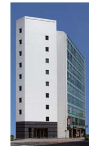
A92 Akihabara SF Building
