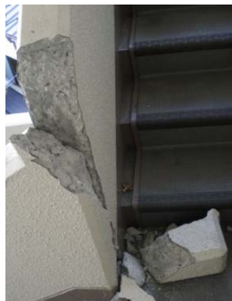
External stairs handrail (4F apart)
