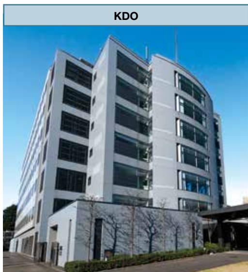
Chofu Center Building (Acquired on June 14, 2019)
