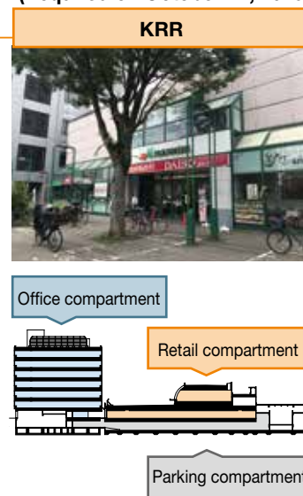
Chofu Center Building (Retail wing) (Acquired on October 24, 2019)
