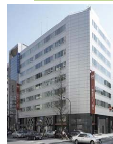
A40 Toranomom Toyo Building
