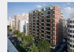
KDX Nagoya Sakae Building
