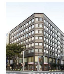
A80 Nagoya Nikko Shoken Building
