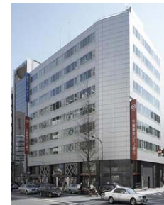
A40 Toranomom Toyo Building
