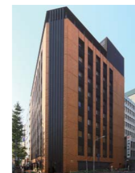
Kyodo Building (Honcho 1chome) Location: Chuo-ku, Tokyo Gross Floor Area: 5,110.45 m 2 Acquisition Price: 4,000 million yen Acquisition Date: November 12, 2010
