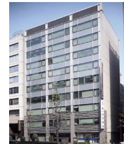
A1 KDX Nihonbashi 313 Building
