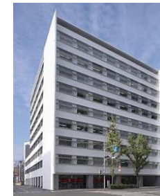
A53 KDX Hakata-Minami Building
