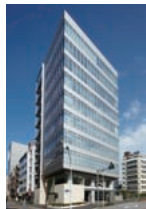
KDX NIHONBASHI 216 BUILDING
