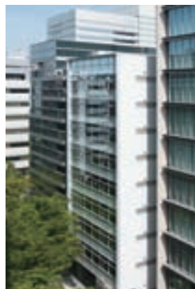
KDX SHIN-YOKOHAMA 381 BUILDING ANNEX TOWER
