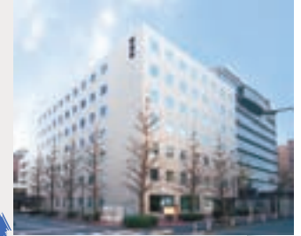
A-37 KDX Ochanomizu Building
