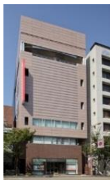
Kanazawa Nikko Building
