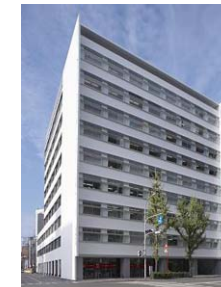
A53 KDX Hakata-Minami Building
