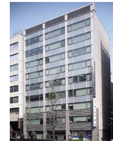
A1 KDX Nihonbashi 313 Building
