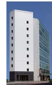
A92 Akihabara Building
