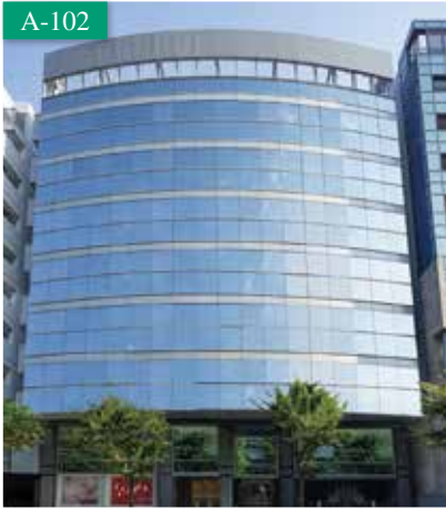
KDX Yokohama Nishiguchi Building
