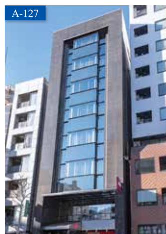
KDX Kanda Ekimae Building
