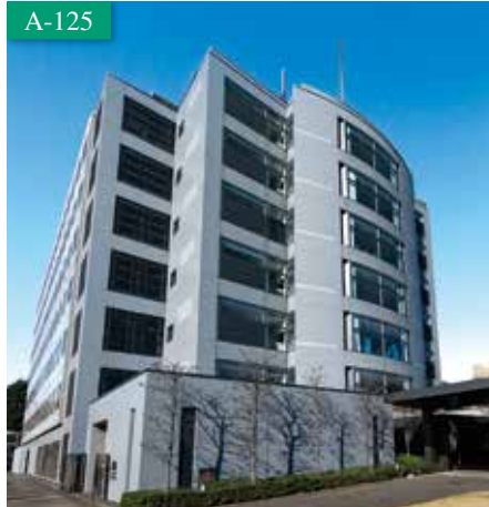
KDX Chofu Building
