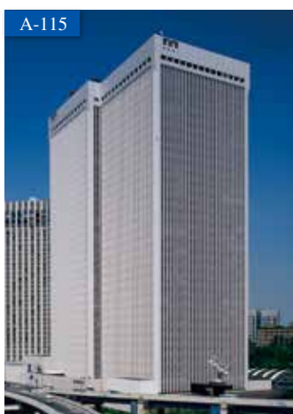
ARK Mori Building (Compartmentalized ownership)
