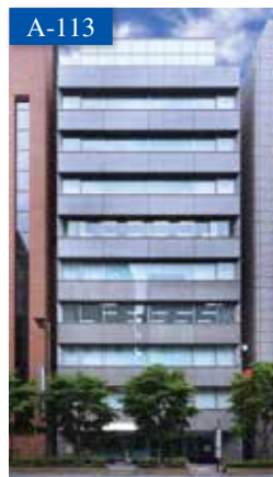
KDX Shin-Nihonbashi Ekimae Building
