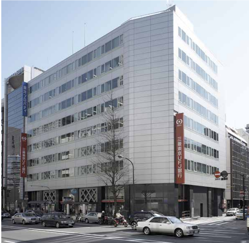
A-40 Toranomom Toyo Building
