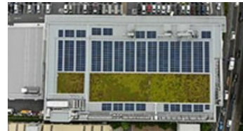
Yumemachi Narashinodai Mall (Power generation capacity: 234.35kW)
