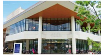
Apita Terrace Yokohama Tsunashima (Power generation capacity: 25.26kW)
