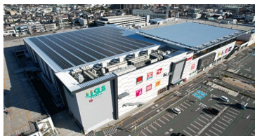
Iias Kasugai (Power generation capacity: 824.76kW)
