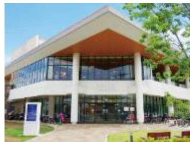
Retail / Apita Terrace Yokohama Tsunashima
